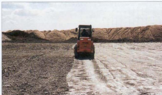
Fig. 4: Levelling und compaction of the clay layer in the catchment area of "Neuer Lugteich"
