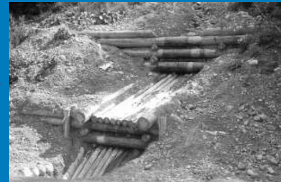
Bolder barriers against erosion gullies
